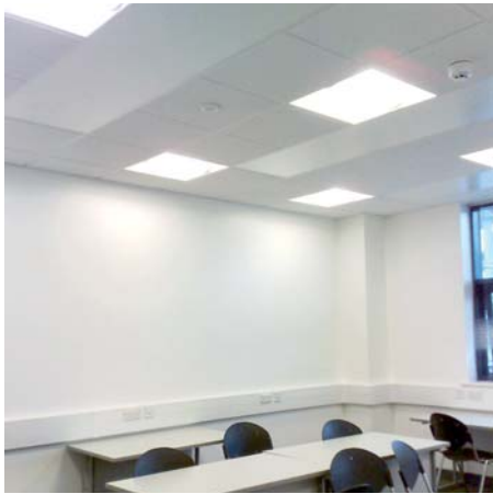
THERMATILE PLUS Radiant Ceiling Panels at Madani High School, Leicester
