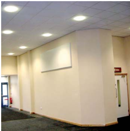
Special close fit wall mounting version of the THERMATILE PLUS Radiant Panels at Doncaster Racecourse and Loughborough Police Station's Custodial Suite (output x 1.2)
