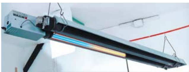
Gas Fired Tube Heaters
